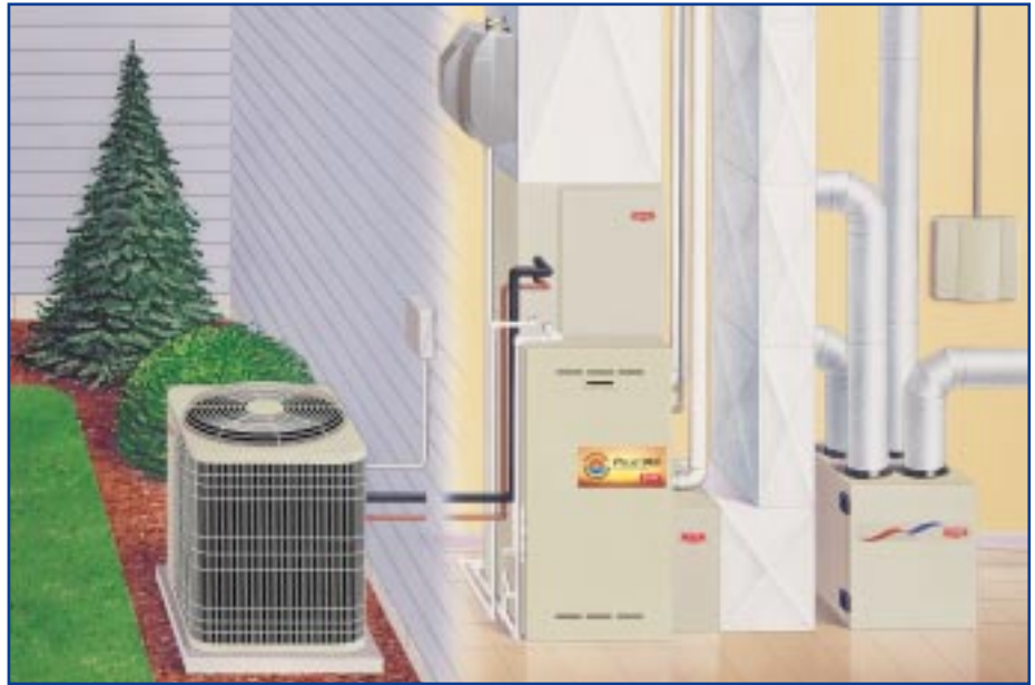
A gas/electric Perfect Humidity System includes a matched combination of a Bryant variable speed furnace, air conditioner, humidifier, and our Thermidistat™ Control.
